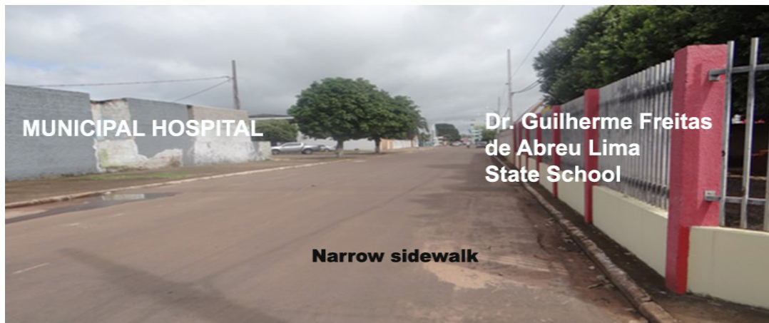
Figure 6 – Narrow sidewalk, Module 1, Cristiane Casquetti Avenue, Juína municipality, MT
